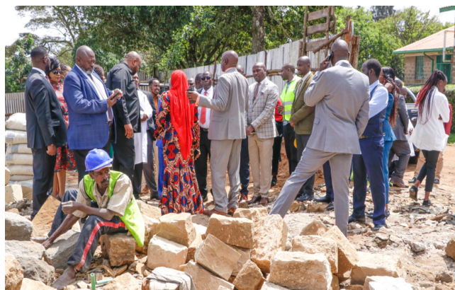
Parliamentary Environment Committee members at Muguga seed facility construction site
